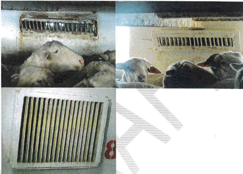
Fig 2-4. Ventilation ducts have been recently enhanced with steel plates within to direct more airflow into the pens and towards the animals.
