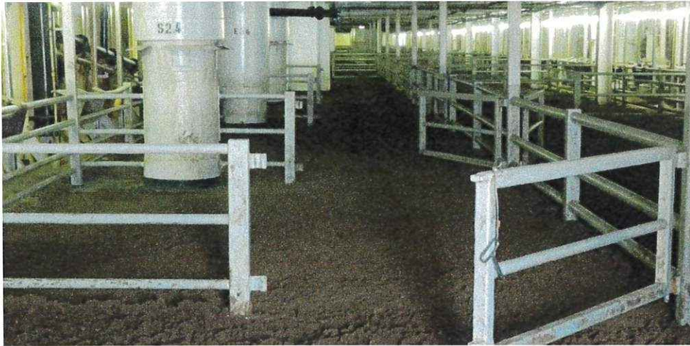
IMG_1589 Column Formation of the Pens Constructed with Pipe Rail Fencing
