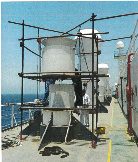
IMG_1722 Ventilation Shaft Maintenance
