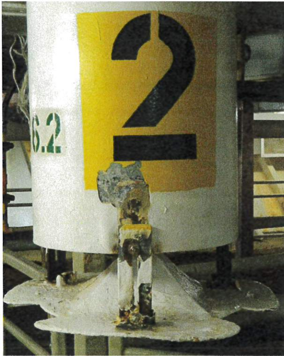
IMG_1760 Adjustment of Ventilation Vent S6.2
