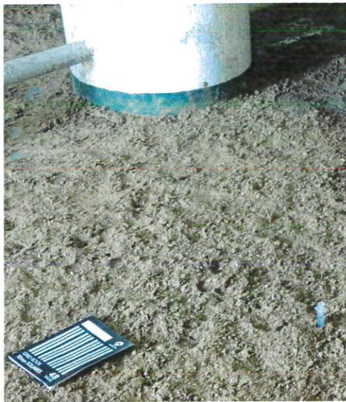
IMG_1564 Depth of Pad Deck 9 Day 16
