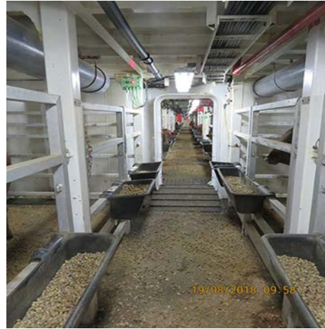
Day 2 Alleyway—no issues identified
